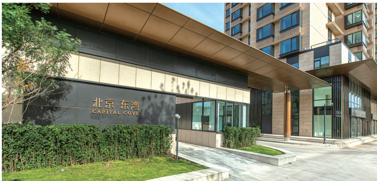
Development project "Capital Cove" in Tongzhou, Beijing
